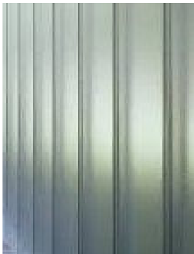
4. Example of 'Glass Planks'. Glazing to ground floor, sports hall
