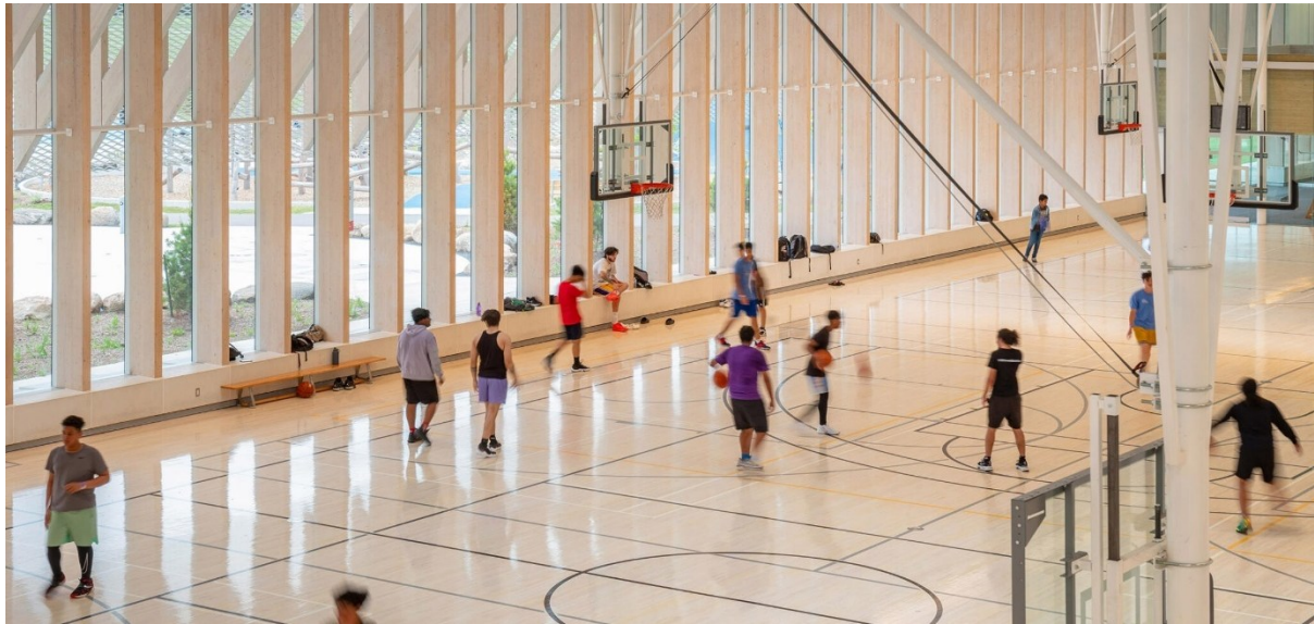
'Glu-Lam' Structure to interior of the sports hall
